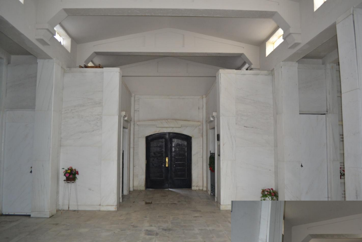
Interior, looking north to front entry in main hall Note the vaulted ceiling and trusses
