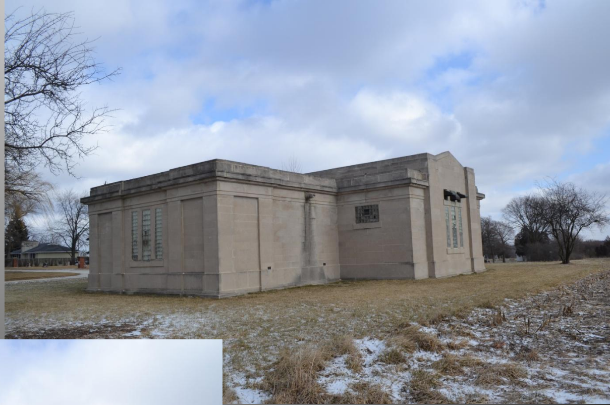
Exterior, looking northeast
